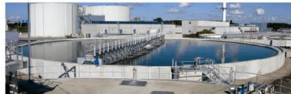
Effluent Treatment & Sewage Plants
